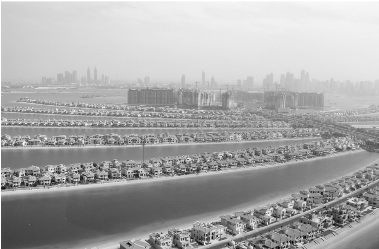
Figure 3. Aerial view of Palm Jumeirah from a helicopter, November 2008; courtesy of Nakheel.
